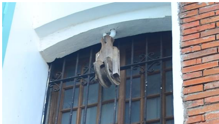
Figure 8. Huge pulley attached to the window brim. Source: Tolentino, R.P.G
