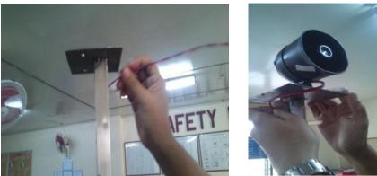
7. Install the siren to the siren holder. Proper wiring should be done to make the siren functional during emergency
