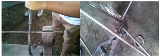
**2.** Layout and construct the steel footings and the boom. Footing must be welded using stainless steel and the boom holds the sensor for a strong foundation of the project
