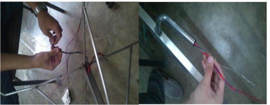
6. Install the wire for the sensor and for the siren. Wires should be inside the boom and must be connected tightly using the soldering iron
